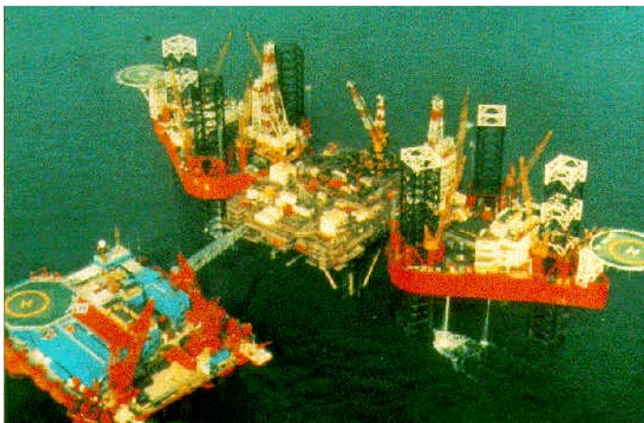
Copper Nickel Sheathing Gas platform - Morcambe Bay - Designed for 40 year life in severe marine environment.
