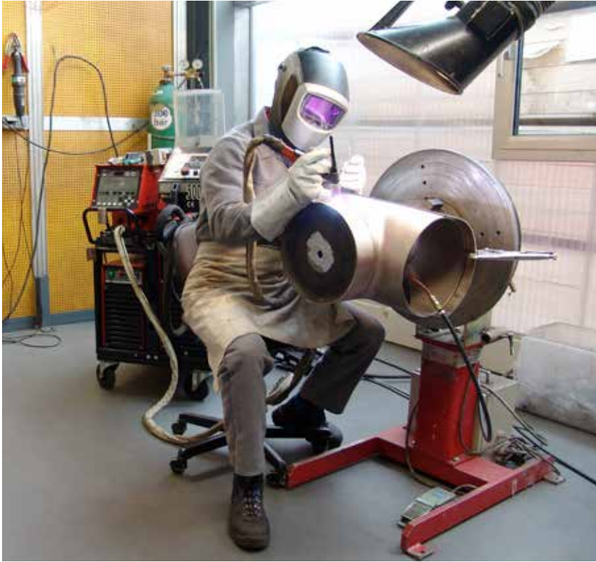
TIG welding 3 rd weld run in joint with pulled T piece (Courtesy Eucaro Buntmetall GmbH)
