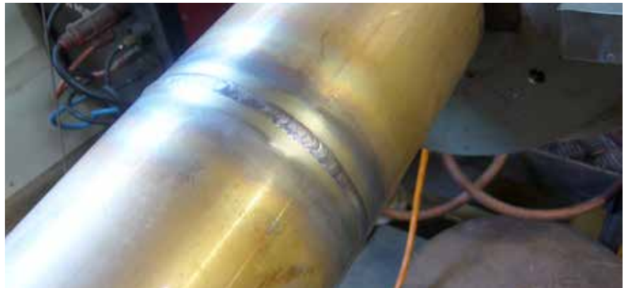
Butt weld showing area which had been cleaned after welding (Courtesy Eucaro Buntmetall GmbH)
