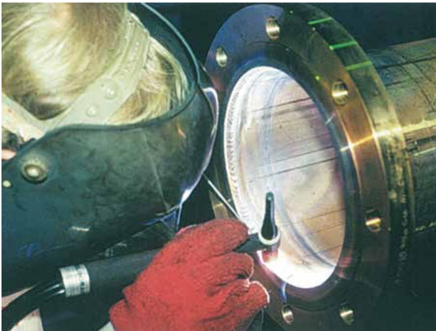
TIG (GTAW) welding a 90-10 copper-nickel assembly
