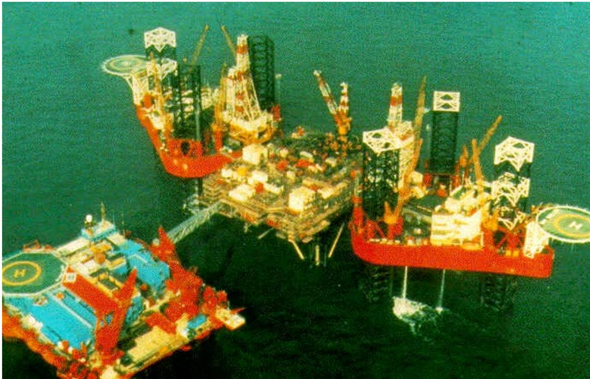
*Morecambe Bay Gas Platform with, copper-nickel alloy cladding in splash zone.
