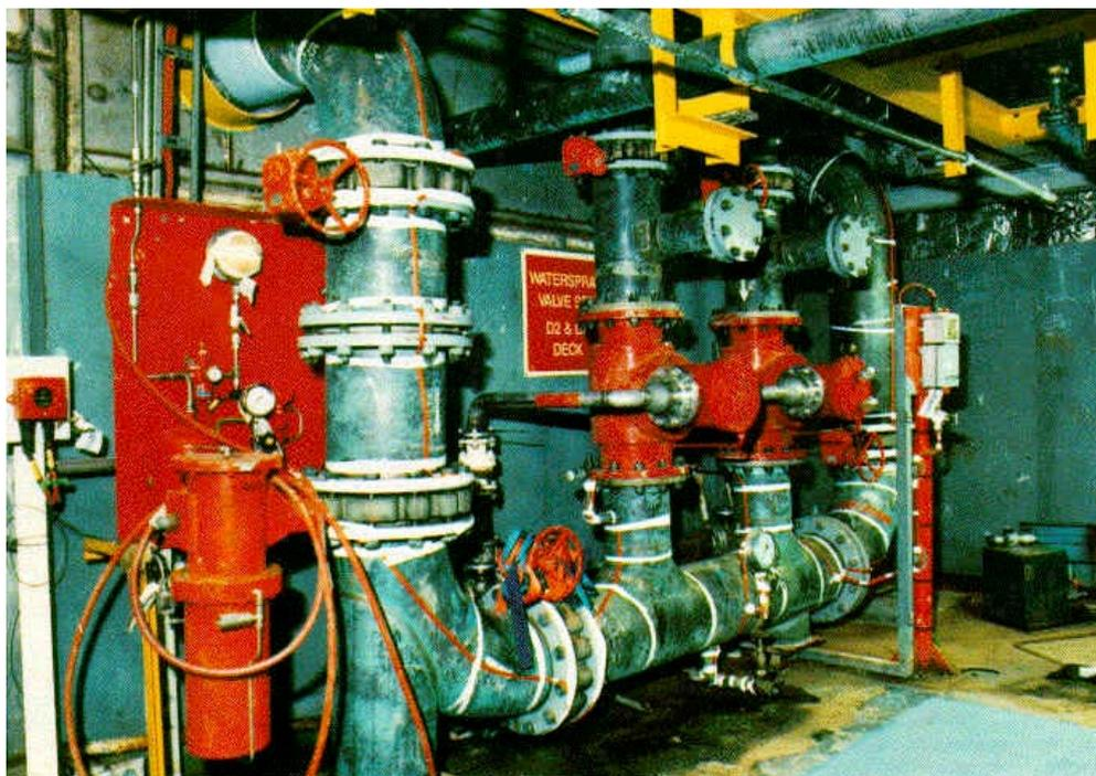
*Copper-nickel alloy pipework on Morecambe Bay Gas Platform.
