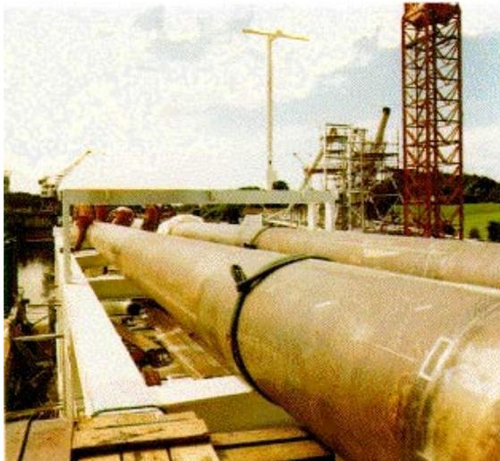
*Figure 2 - 711 mm O/D CuNi10Fe1Mn pipework in Frigg. TCP2 compression module at Grinstad Norway (photo: IMI Dreh).*
