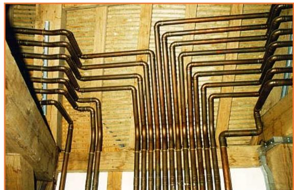
To achieve the same flow rate as copper, certain other materials will need to have a larger sized tube for the same bore size that compromises the aesthetic appearance of the pipework.
