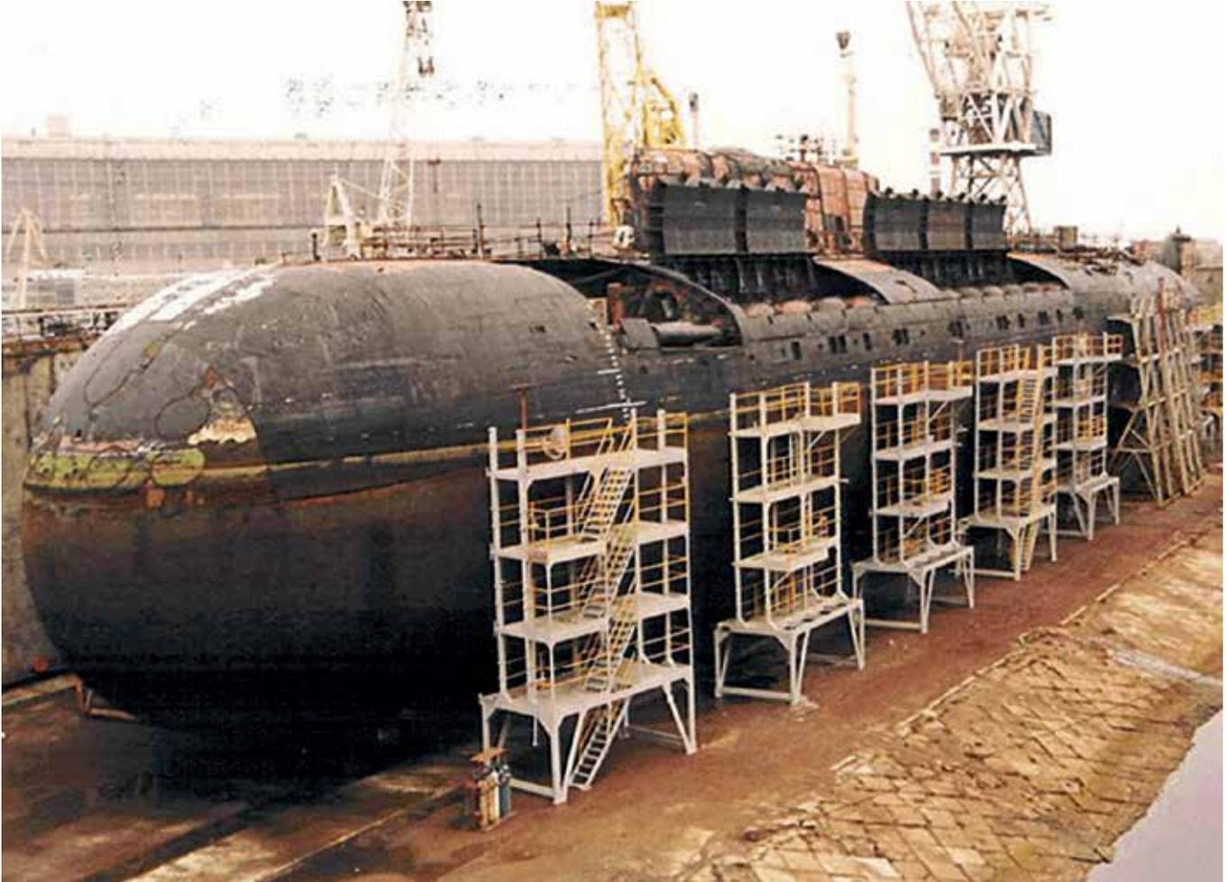
Figure 17 - Dismantling Oscar 1 Class Submarine (Courtesy Keel Marine Ltd)
