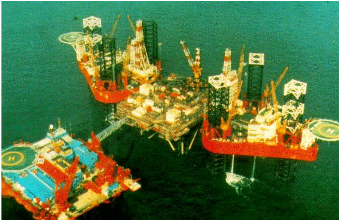
Morecambe Bay Gas Platform with, copper-nickel alloy cladding in splash zone. [photo: British Gas Corporation]
